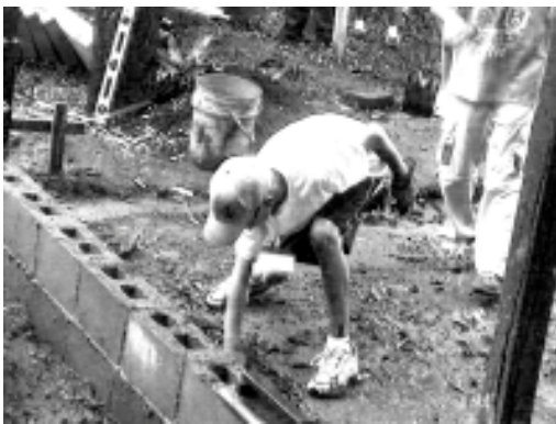
Greg Drosky helping to build the gazebo wall.
