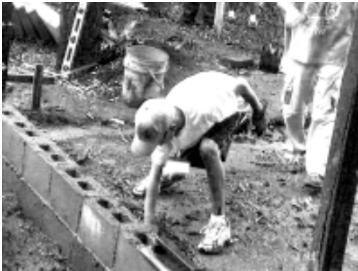
Greg Drosky helping to build the gazebo wall.
